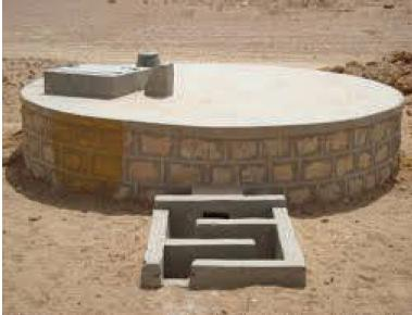
**Backfilling:** Backfill the excavation around the tank with soil or sand, compacting each layer as you go.
